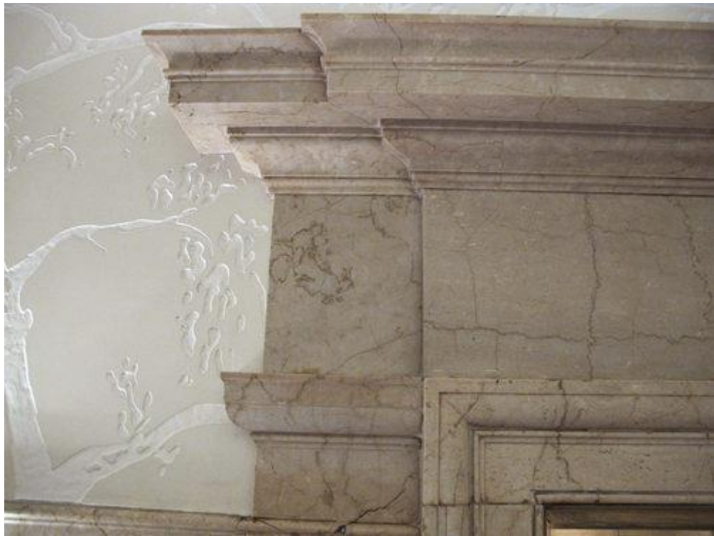
The wall is etched around the front door.
